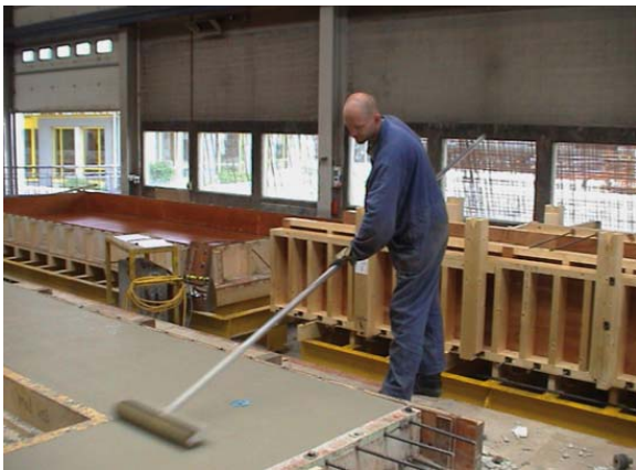
Figure 7: Finishing the surface.
