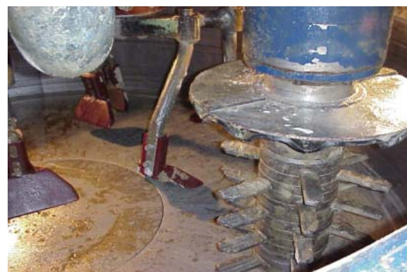
Figure 3: Wirbler and scraper installed
