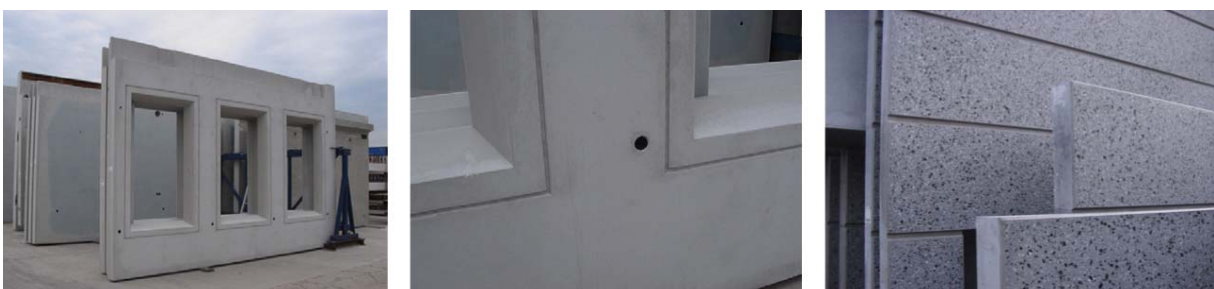
Figure 8: Appearance SCC
