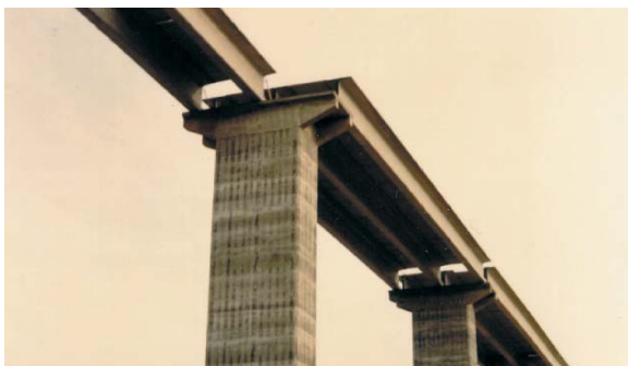
Fig 48: Precast crossheads on site cast piers
