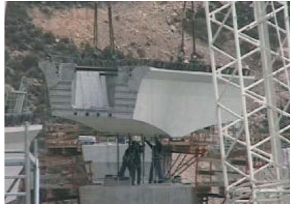
Fig. 17: Piece in cantilever over the pier
