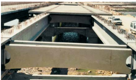
Fig. 32 & 33: Precast deck slabs of full thickness
