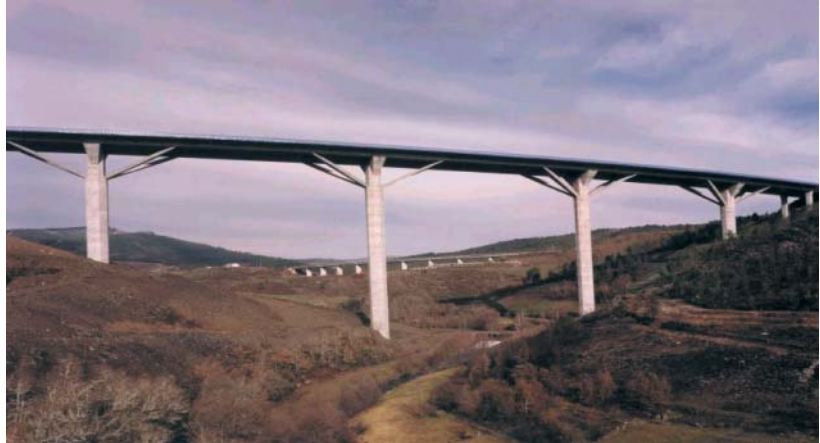
Fig. 18 & 19: Bridge with spans supported on diagonals, during construction & complete
