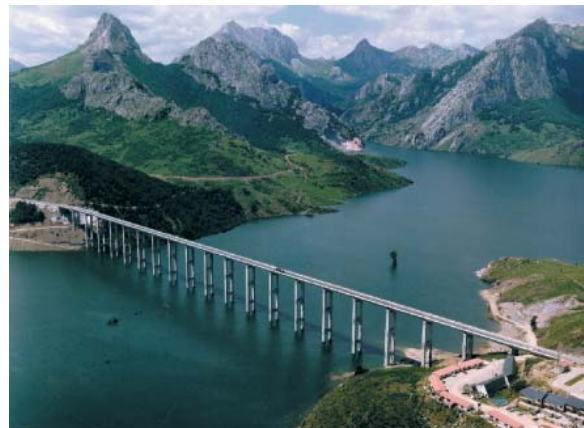
Fig 50: Precast bridge with piers 65 m tall
