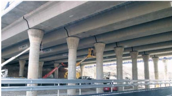
Fig. 26: Bridge with decks of U-beams
