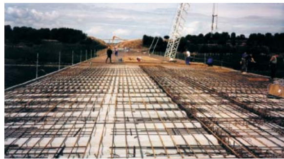
Fig. 31: Upper reinforcement mesh placed on partially precast slabs of bridge decks
