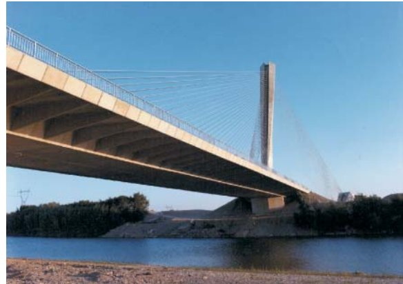
Fig. 9: Ebro bridge – Navarra motorway
