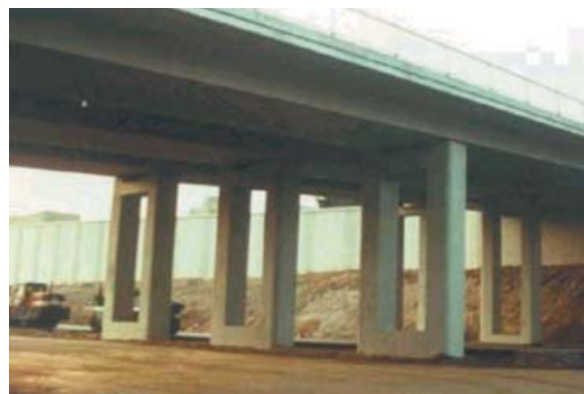
Fig. 51: Portal frame piers of reduced height prefabricated in only one piece
