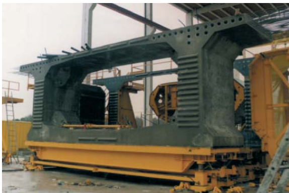
Fig. 36: Segment of partial transversal section
