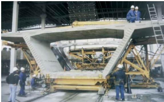
Fig. 35: Segment of full transversal section at the precast plant
