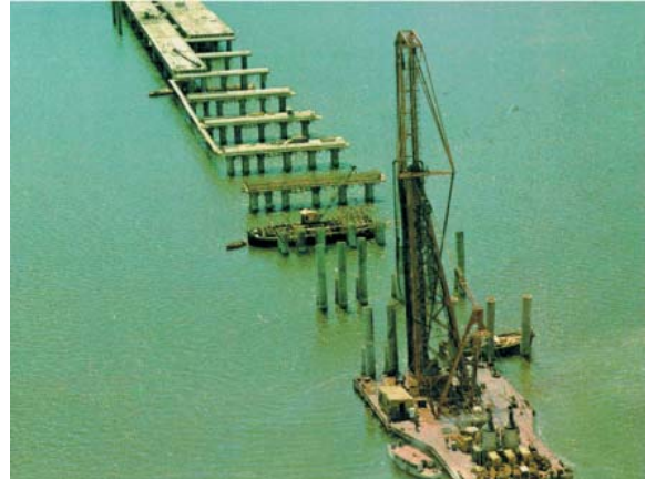
Fig. 2: Bridge over Tinto River
