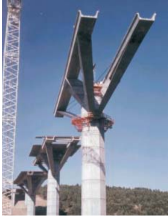
Fig. 18 & 19: Bridge with spans supported on diagonals, during construction & complete
