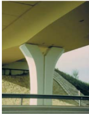
Fig. 45 to 47: Piers of independent columns with simple and double capital
