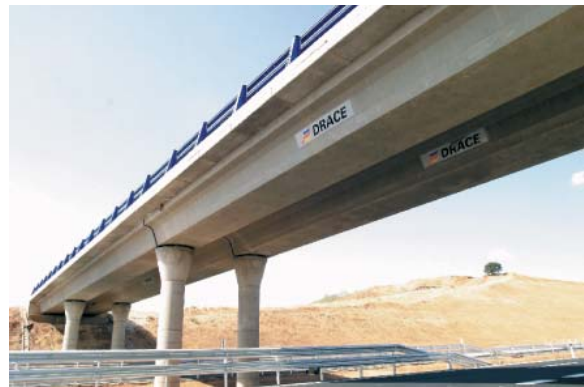
Fig. 11: Precast bridge with U beams deck
