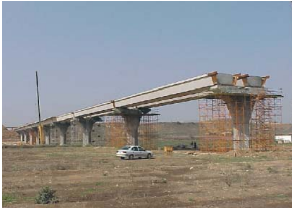
Fig. 13: High Speed railway bridge with hyperstatic continuity
