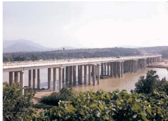
Fig. 4: Ebro bridge – Tarragona motorway
