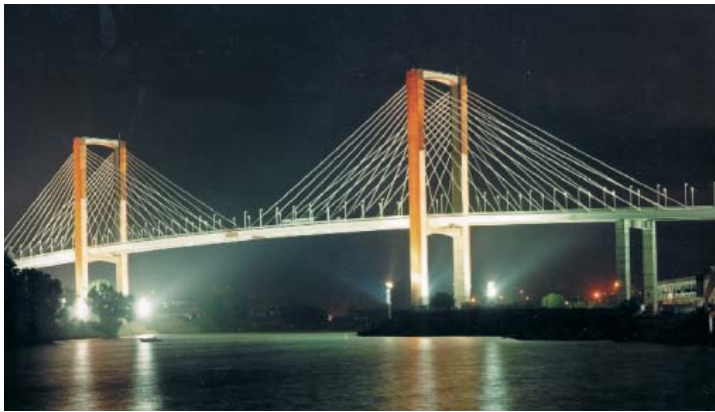
Fig. 20 & 21: Cable stayed bridge with precast concrete deck, complete & during construction
