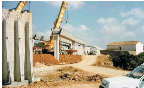
Fig. 44: Abutments of cantilever counterfort elements
