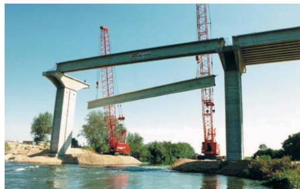
Fig. 24: Bridge with decks of I-beams
