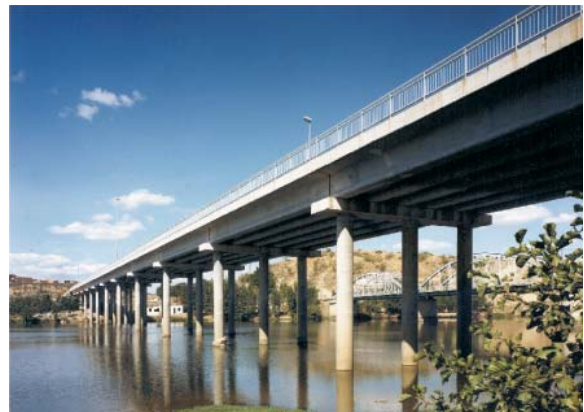
Fig. 10: Precast bridge with I beams deck
