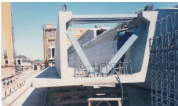
Fig. 28 & 29: U-beam for railway bridge with longitudinal joint to form a triclular box
