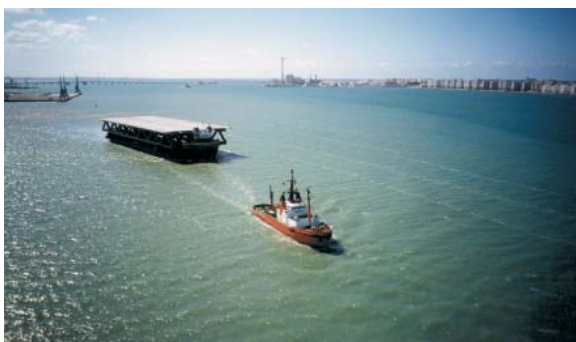
Fig. 41 & 42: Oresund bridge: Transport by sea and installation on piers by a very big crane
