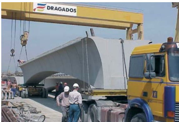
Fig. 14: Transport of variable height U beam
