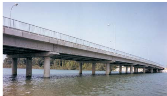
Fig. 49: Frame piers with Raymond piles
