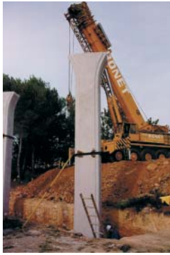
Fig. 45 to 47: Piers of independent columns with simple and double capital
