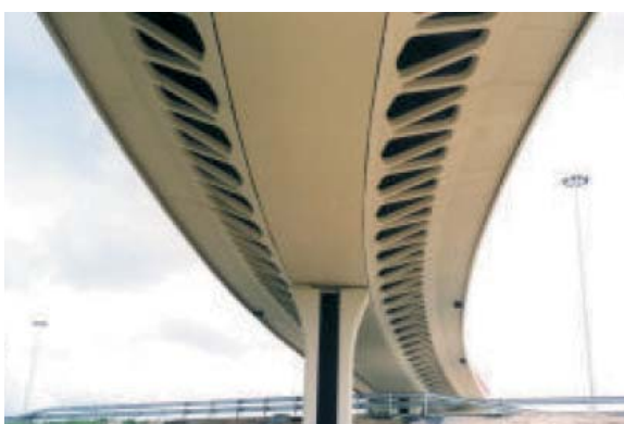
Fig. 16: Diagonals of complex shape
