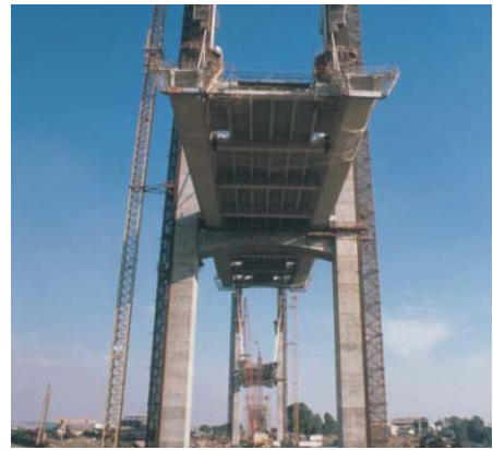
Fig. 20 & 21: Cable stayed bridge with precast concrete deck, complete & during construction
