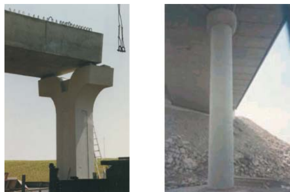
Fig. 12: Precast bridges with mono-beams
