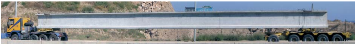
Fig. 25: Transport of a large I-beam by road
