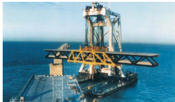
Fig. 41 & 42: Oresund bridge: Transport by sea and installation on piers by a very big crane
