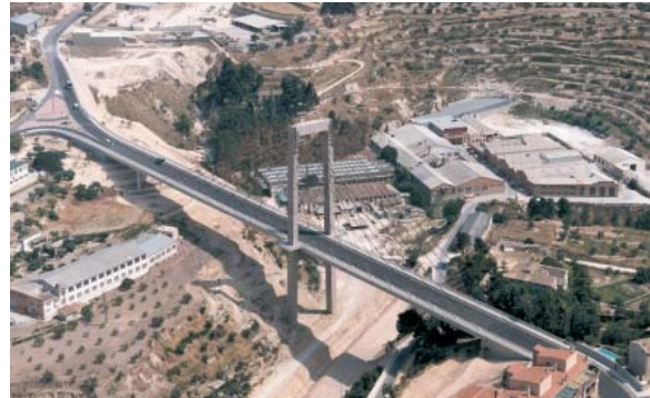
Fig. 38: Precast cable stayed bridge deck
