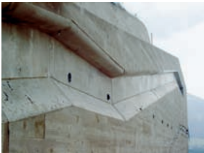
Station Hungerburg – Betondetails
