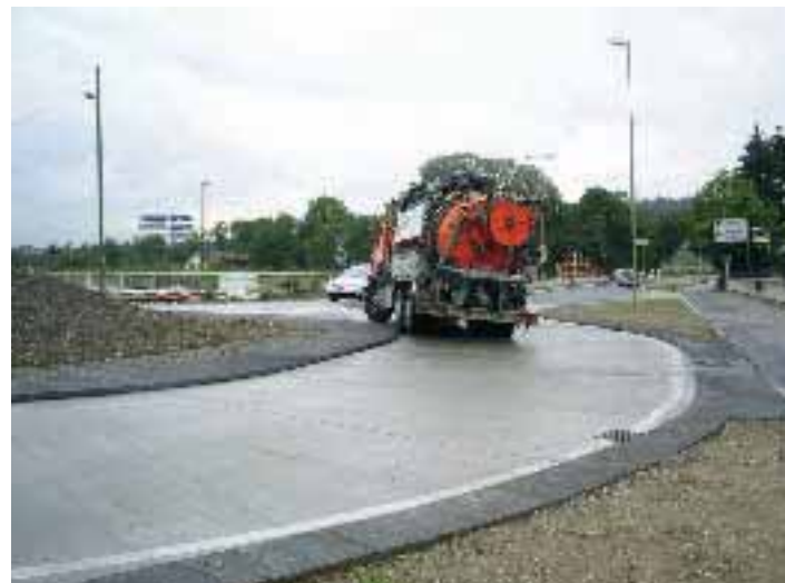
Neftenbach ZH, Randabschlüsse in Beton
