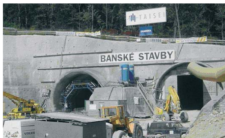
Picture 6 – Tunnel Sitina – Construction of south tunnel face
