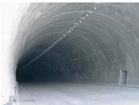
Picture 5 – Concrete road in tunnel Horelica
