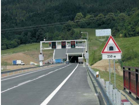
Picture 2 – Tunnel Branisko – West tunnel face
