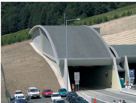
Picture 4 – East tunnel face of tunnel Branisko
