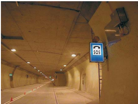
Picture 3 – Concrete road in tunnel Branisko
