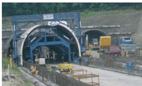
Picture 8 – Construction of second lining in north tunnel face
