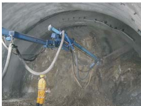
Picture 7 – Tunnel Sitina – shotcreting of primary lining
