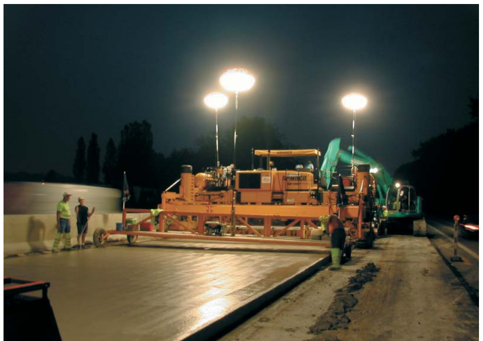
Figure 3: Slip form paver at night on the E40
