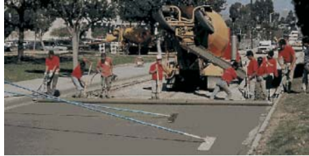
Figure 11: Roller Screed (Revolving Tube) paving technique for low volume roads
