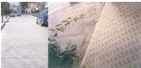
Figure 3: the concrete block pavement in Recoaro after 11 years of service.
