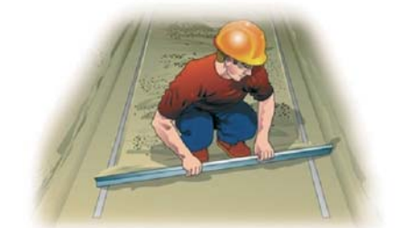
Figure 14: laying the sand roadbed of a concrete block pavement
