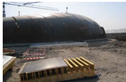
Abb. 27: Doha Beach Villa, Qatar
