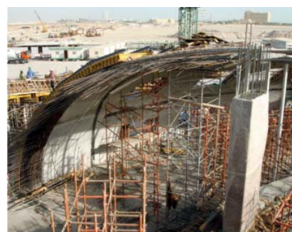
Abb. 28: Doha Beach Villa, Qatar
