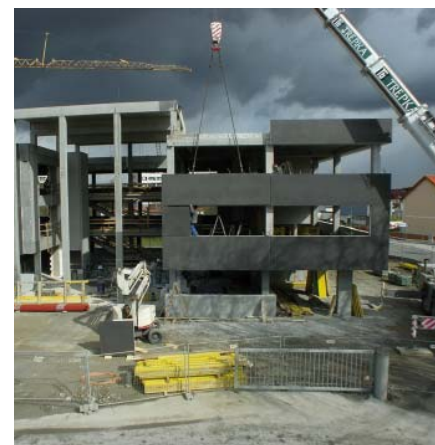
Abb. 6: Montage Sandwichwand
